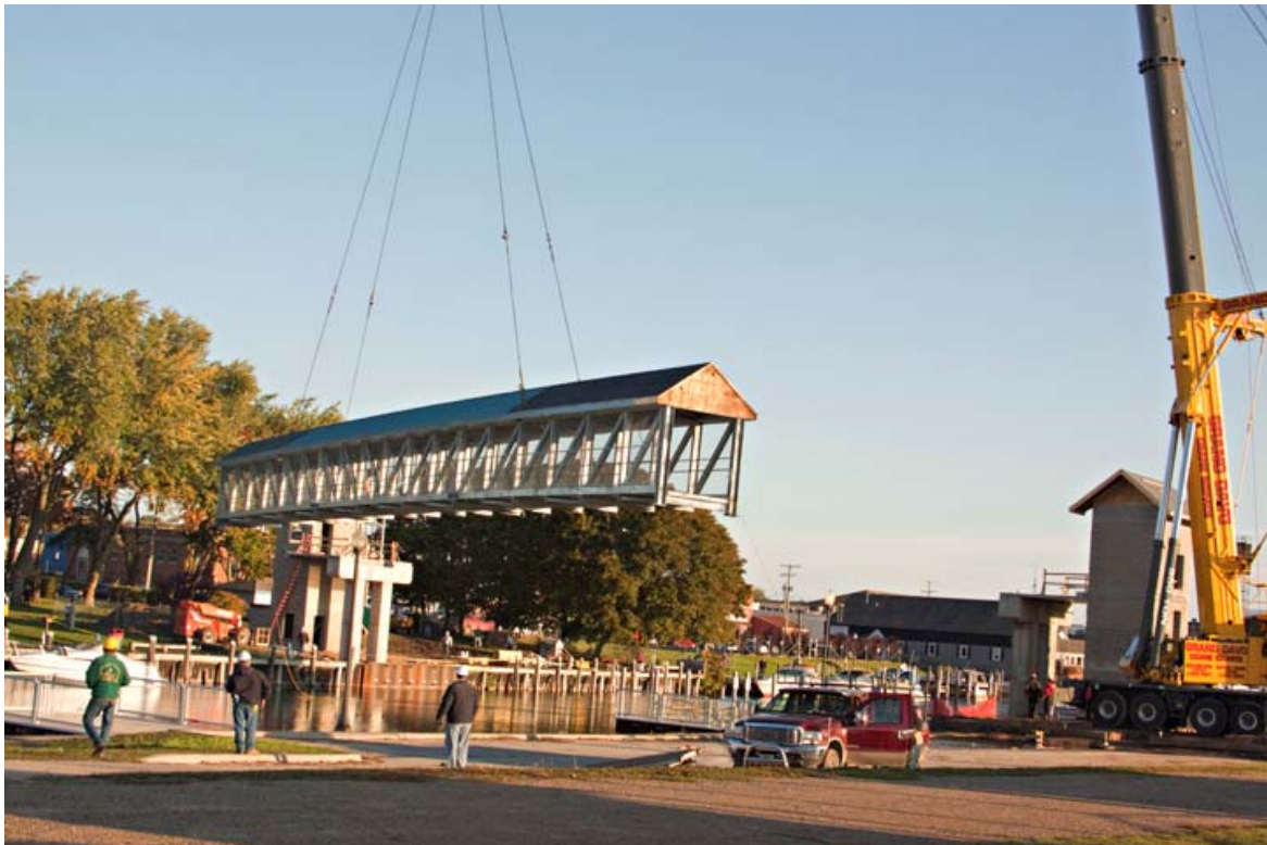
Footbridge placed over Cheboygan River, Oct. 8
